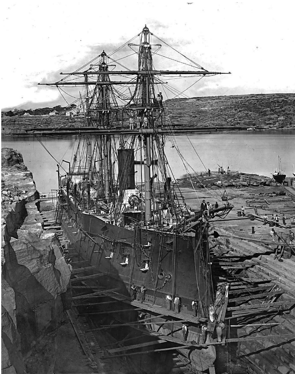
The French iron-clad Atalante in Fitzroy Dock, Cockatoo Island, in August 1873, with Cuthbert's men at work on the hull and armour plating.
